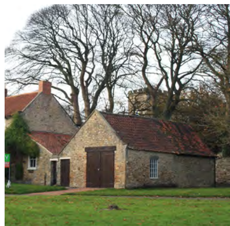
Boundary walls and outbuildings are numerous, adding great historic integrity to the area
